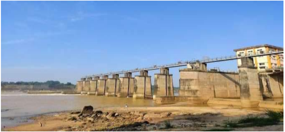
Fig-4: Tarkera Intake Water Structure On The River Brahmani
